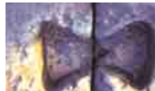
Imprint of metal clamp on stone structures at Angkor Wat, Cambodia
